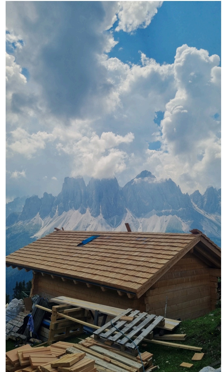
The cold shell for the new hut.
